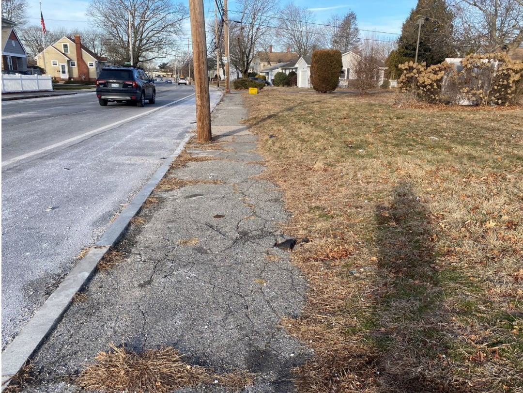
Figure 3: Sidewalk in front of Site (Photo Taken on 1/16/2025)
