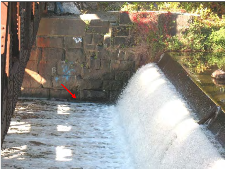
Photo 21. Omega Pond Dam. Right dam abutment from left abutment wall. Note open masonry joints, missing stone step at bottom (arrow) and vegetation.
