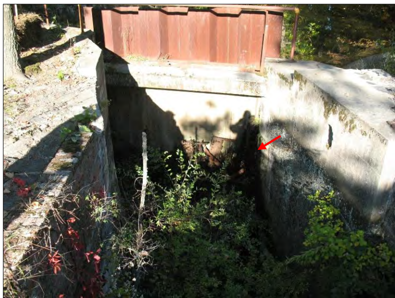
Photo 13. Hunt's Mill Dam. Downstream view of abandoned headrace closure wall leaking at left corner (arrow).
