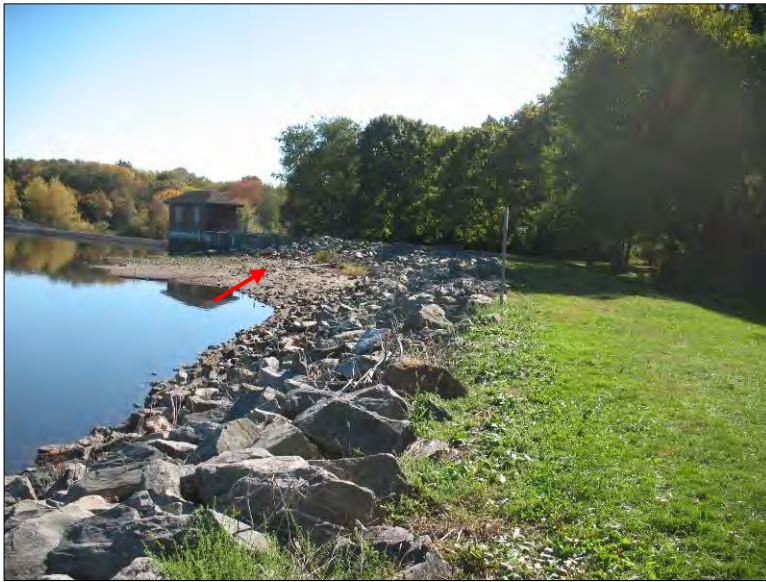
Photo 7. Turner Reservoir Dam. Right dike looking toward gatehouse. Note upstream slope area with missing riprap (arrow).
