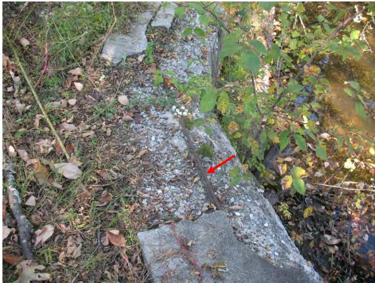
Photo 16. Hunt's Mill Dam. Deteriorated concrete with exposed reinforcement on top of upstream retaining wall (arrow).
