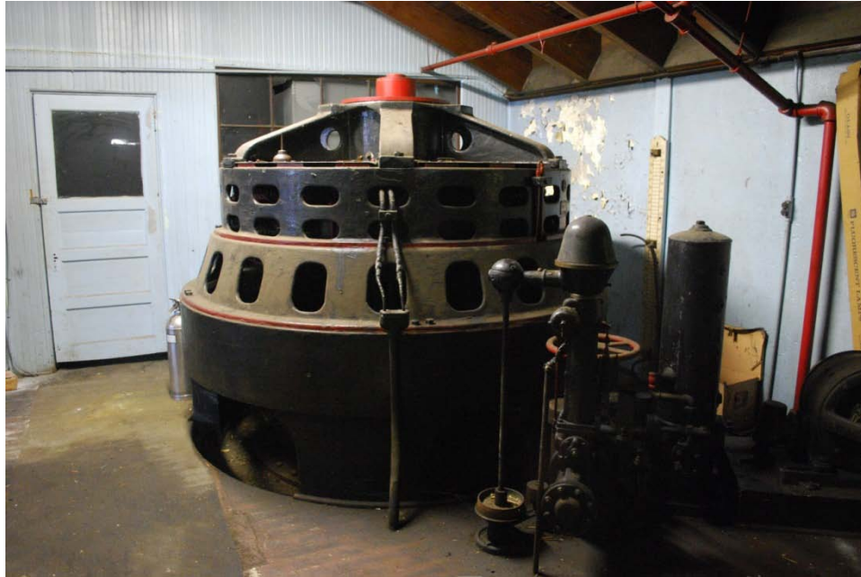
Figure 4. Existing Hunt's Mill Generator and Governor
