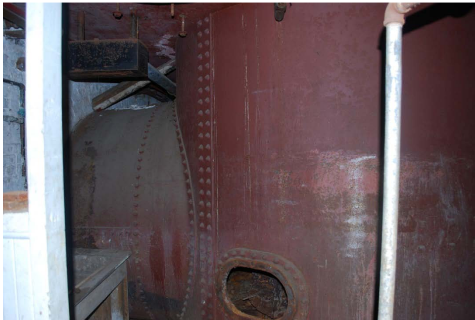
Figure 5. Steel penstock and Vertical Pressure Case
