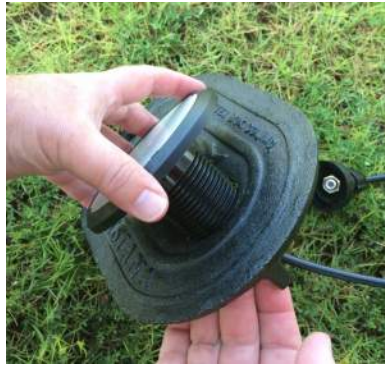
Figure 22 – Inserting Antenna into Pit Lid
