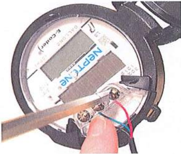
Figure 3: Wiring with Proper Color Wires
