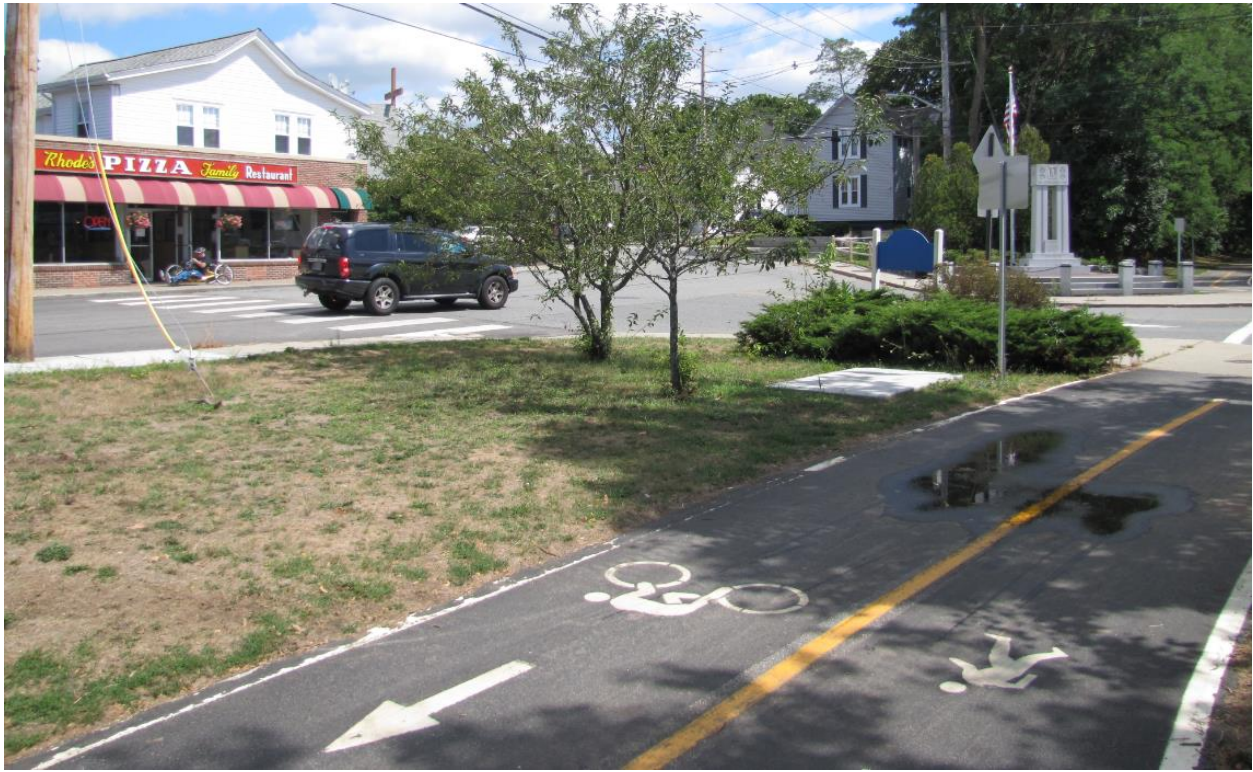
Looking South at Path Entering Turner Ave. / Riversdie Sq.
