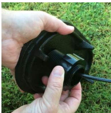
Figure 24 – Securing the Locking Nut
