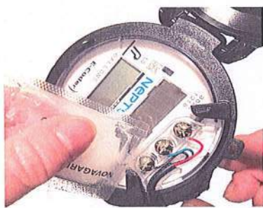
Figure 5: Applying Compound
