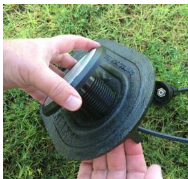
Figure 22 – Inserting Antenna into Pit Lid
