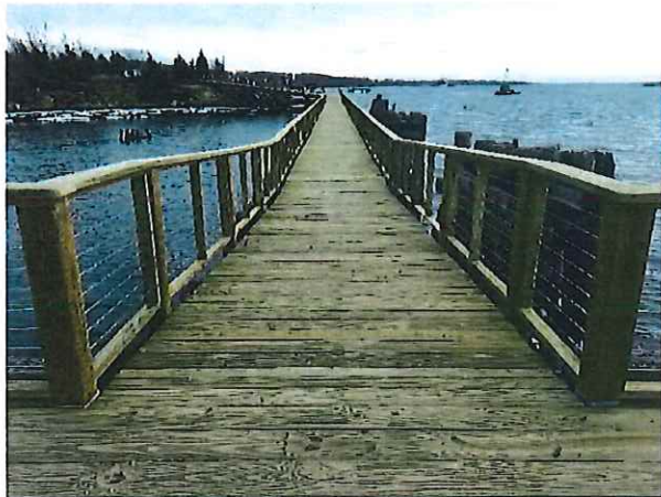
Figure 3 View from viewing deck toward Kettle Point
