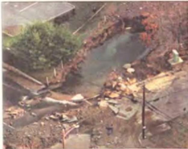
CRATER: The 102-inch underground rupture of the transmission of Metropolitan Water Park, right, and Clarksburg.
