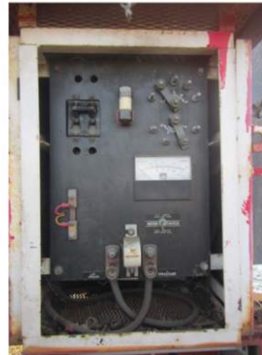
Photo No. 1: Providence Rectifier
