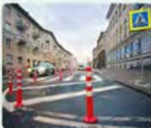
Transverse Striping and Flex-Post/Bollard Curb Extensions Photo courtesy of Ticky Sherkikote Stock
