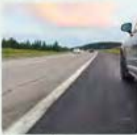
Paved Shoulder Photo courtesy of BakerAdobe Stock
