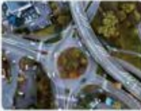
Corridor Access Management Photo courtesy of Song_about_summer/Adobe Stock
