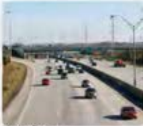
Median Barriers Photo courtesy of Kenneth Sponser/Adobe Stock
