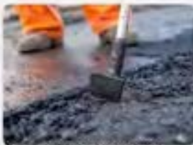
Pavement Friction Management Photo courtesy of Artificion/Adobe Stock
