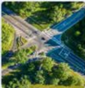
Vegetation near Intersection Photo courtesy of ostrom/Adobe Stock
