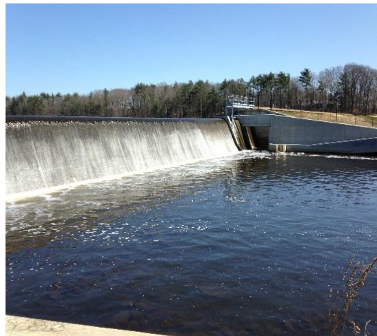
Photo 9. Turner Reservoir Dam. Photo: Wayne Barnes
