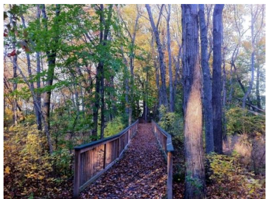
Photo 2. Turner Reservoir Trail raised walkway segment. Photo: Wayne Barnes
