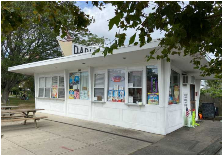
240 Bullocks Point Avenue, front (west elevation)
