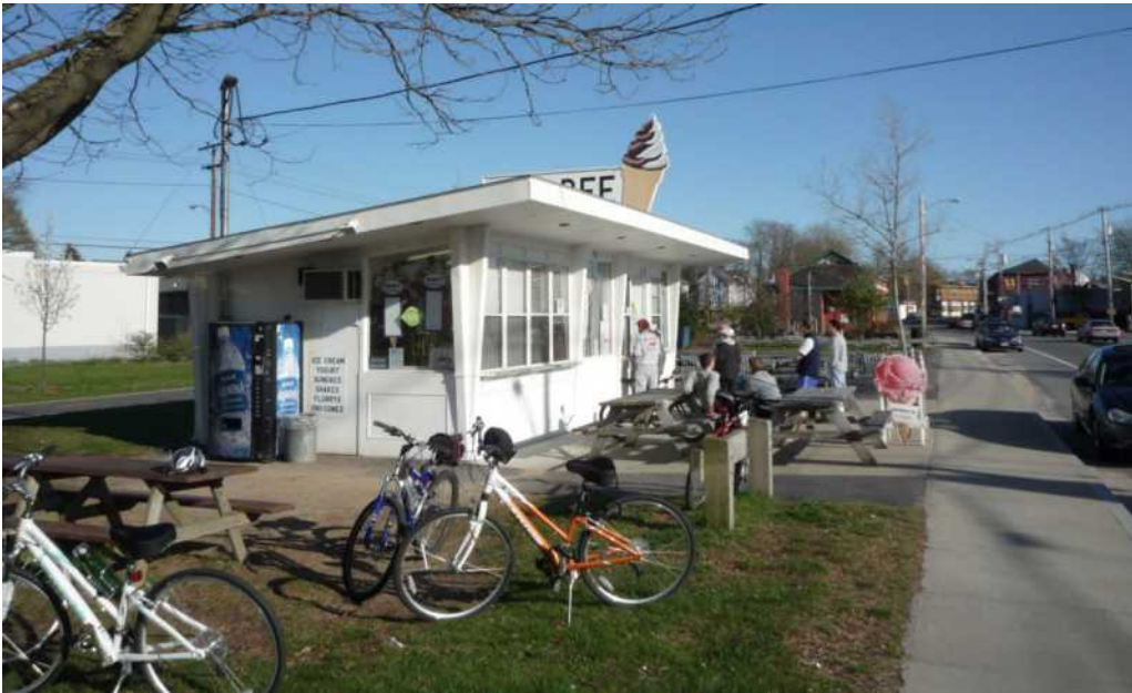
Side (north) elevation, facing south
