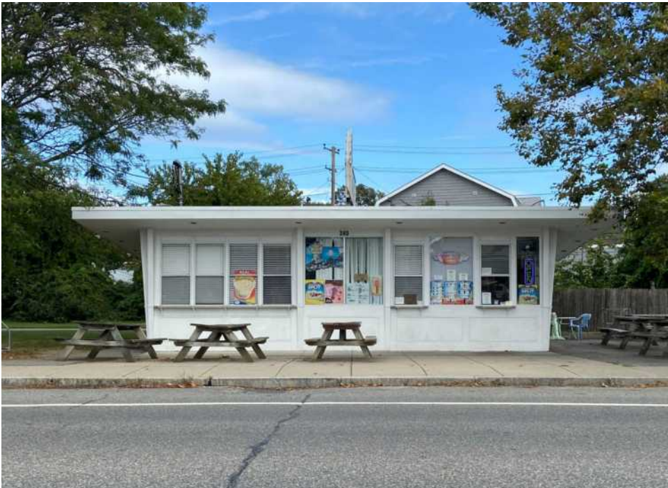
240 Bullocks Point Avenue, front (west elevation)
