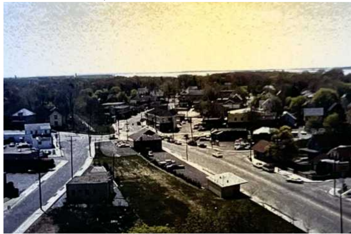
Photo of Bullocks Point Avenue, showing the depot, the demolished Bee-Hive gift shop, and Dari-Bee, Date is unknown. Source: From the East Providence City Hall Picture Records
