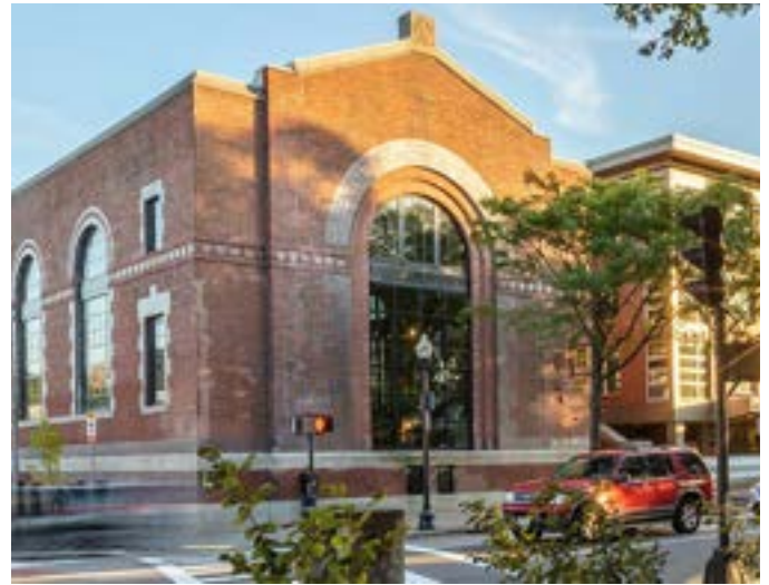
Figure 1.15 Revitalized 1911 Roslindale Substation. Source: Historic Boston
