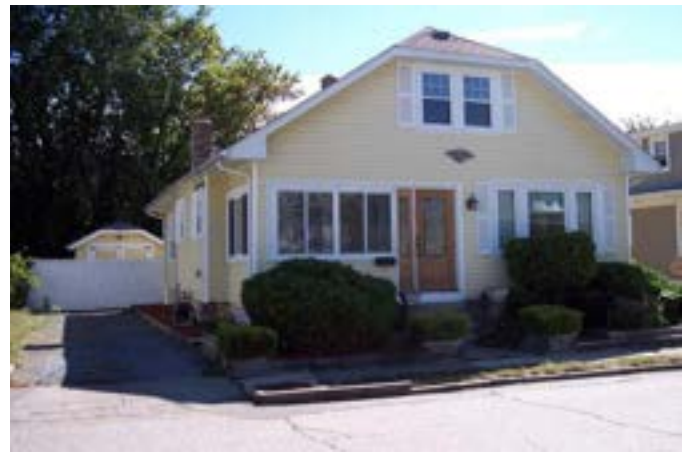
Figure 3.25 Elinora House Rehabilitation Project, Before.
