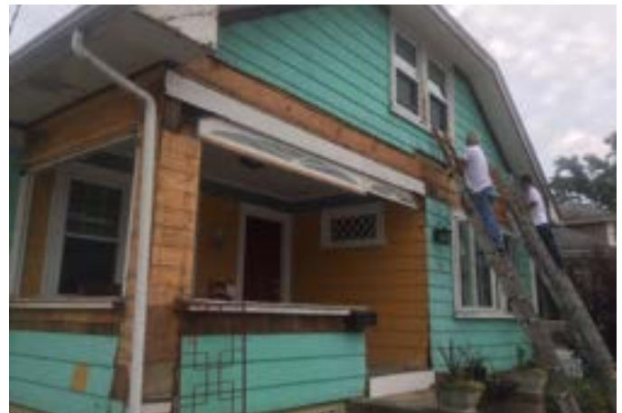
Figure 3.26 Elinora House Rehabilitation Project, Vinyl Removal.
