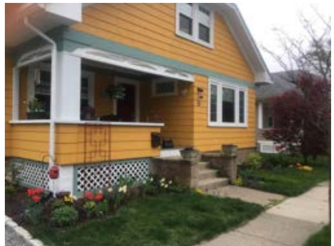
Figure 3.27 Elinora House Rehabilitation Project, After.
