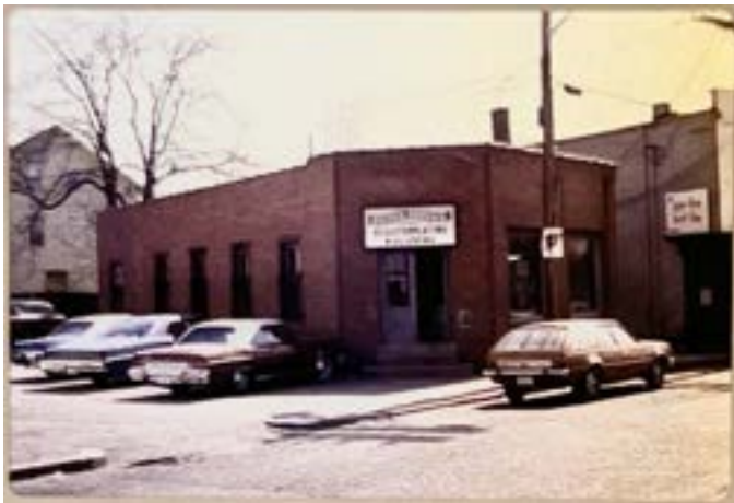
Figure 3.20 Riverside Post Office. c.1970.
