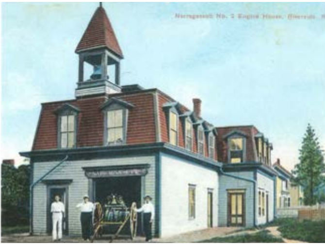
Figure 3.4 First Riverside Fire Station built c. 1880.
