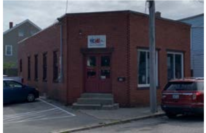
Figure 3.23 Old Riverside Post Office, Present Day.
