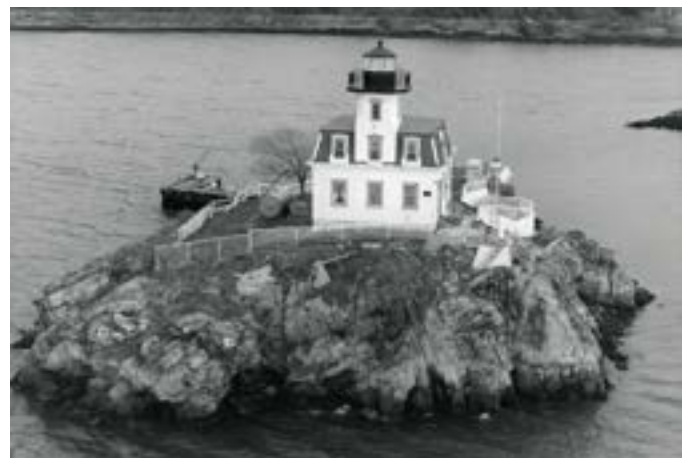
Figure 3.17 Pomham Rocks Light Station.
