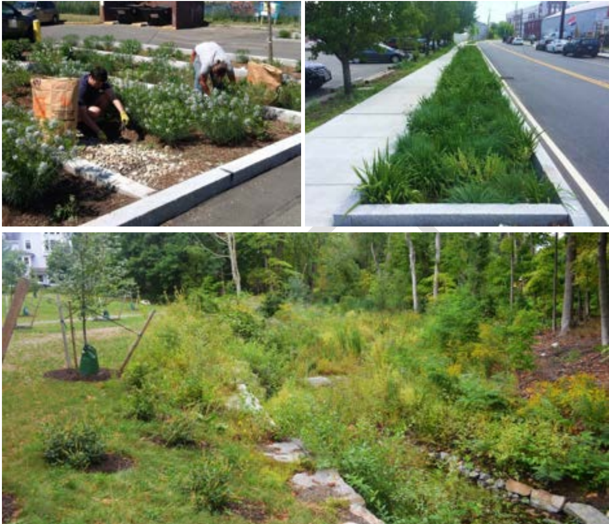
NBS installations are diverse in function and size and can be incorporated into parking lots, along streets and sidewalks, and blended into larger landscaped areas.
