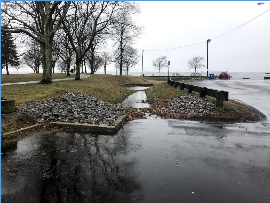
Sabin Point sand filter treats stormwater runoff before flowing into the Bay
