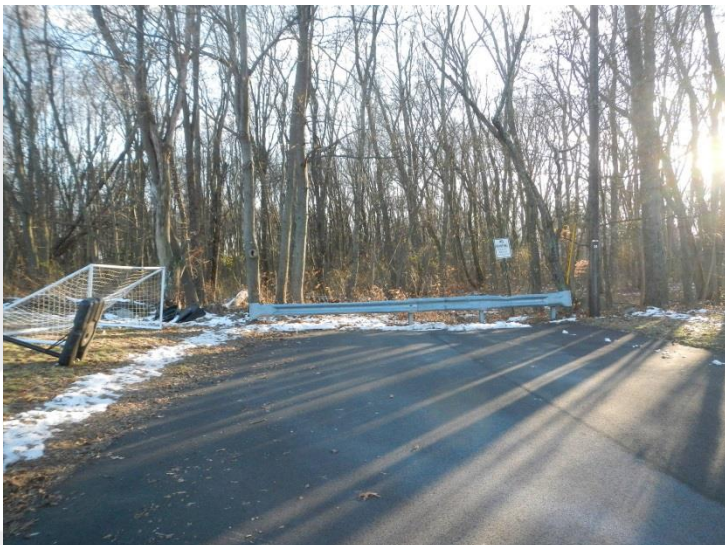
Looking South from Elder Street
