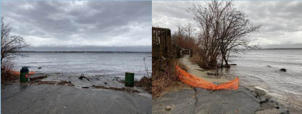
Storm surge at Beach Road after a storm, January 22, 2021.
