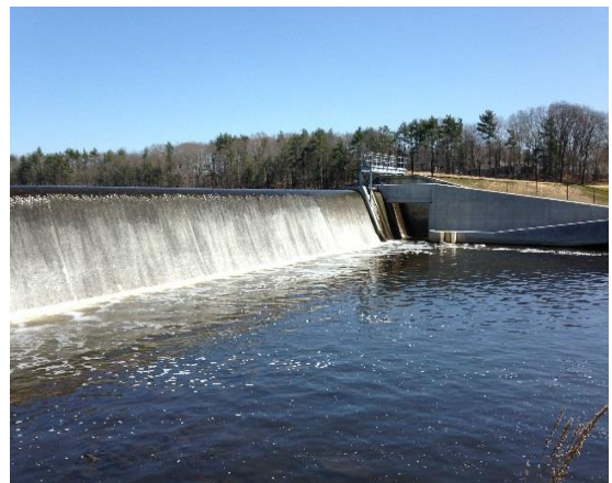
Photo 13. Turner Reservoir Dam. Photo: Wayne Barnes
