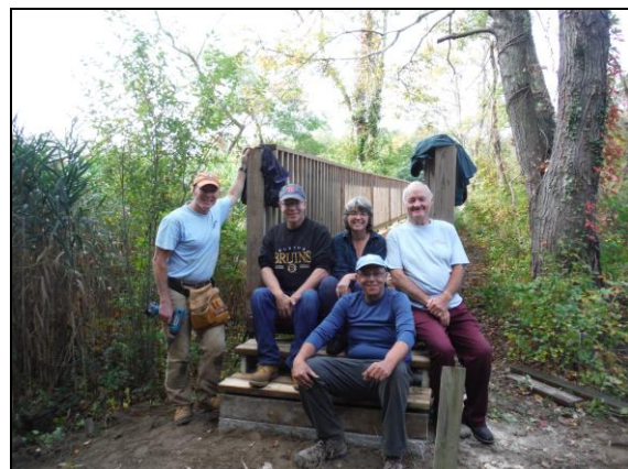
Wetland Boardwalk Stairway Completed
